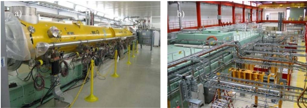
**Figure 2:** Photographs of an installed cryomodule (left) and the shielded tunnel and installed rf and power supply infrastructure (right).
